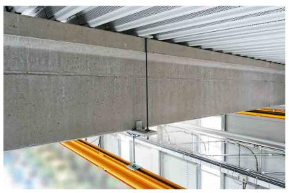
The threaded rods at the side are variable in length and enable even large truss heights to be used. Depending on the ceiling construction, embracing brackets can also be mounted on the ceilings on top of the building trusses.
